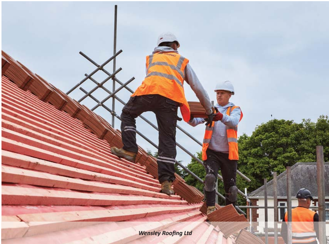
Arcas Building Services Ltd - Inn Collection Group, The Stables, Whitby
