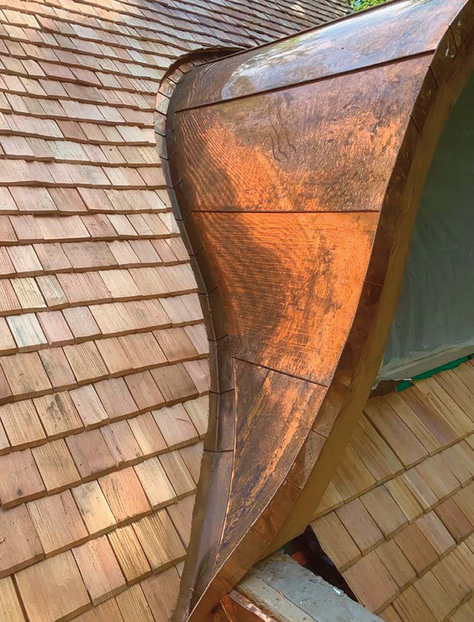
Private House, Longhorsley, Northumberland – Wensley Roofing Ltd
