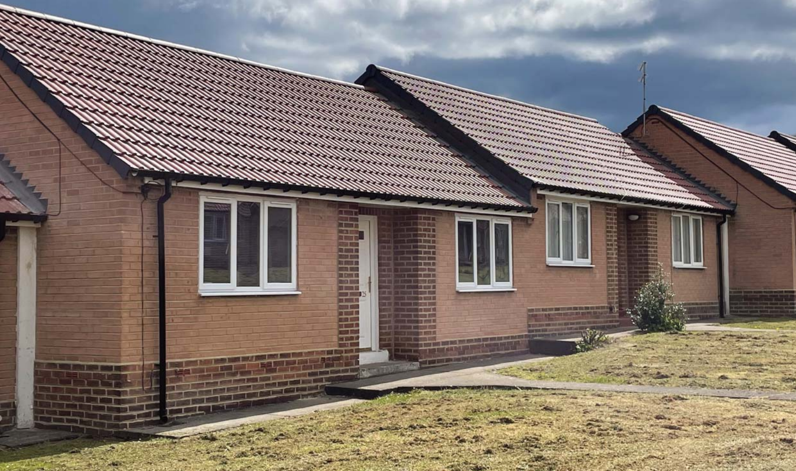
Re-Roofing Scheme Seaham/Horden, Co. Durham – Springs Roofing Ltd
